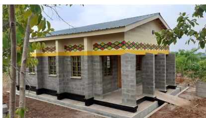
Nursery block seen from the side
