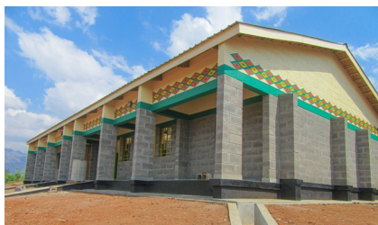
Block 4 of classrooms
